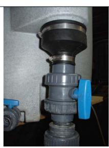
16)On pump fed installations push the adjustable collar on the exit stand pipe to its lowest setting
