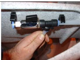
15)Connect the new back wash air tube to the other side of the air valve.
