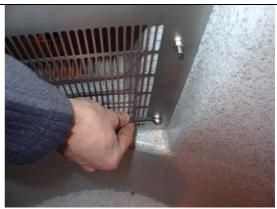
11)Using the template supplied drill two 4mm holes in the side of the inner drum.
