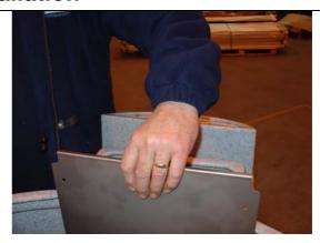
2) Remove the existing exit "D-Plate" by unscrewing and withdrawing the two retaining screws. Ensure that the sealing washer on each screw is not lost as these will be required to ensure a leak proof installation. Set aside all fixings as these will be required later.
