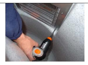
10) Fit and tighten the two lower fixings using the screws, washers and nuts supplied. (Ensure that the sealing washers are fitted on the outside of the tank under the heads of all screws).
